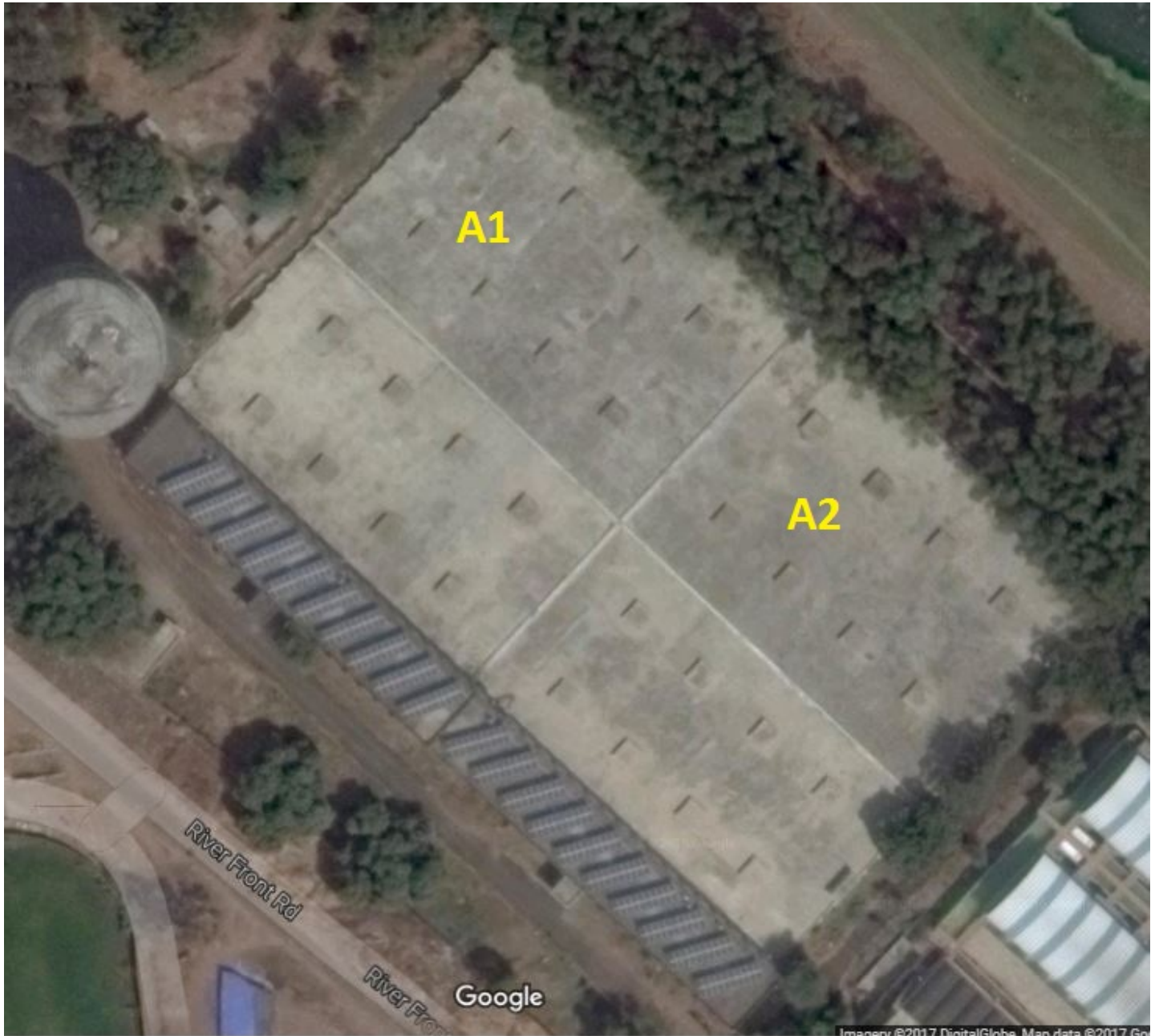
Katargam Water works
