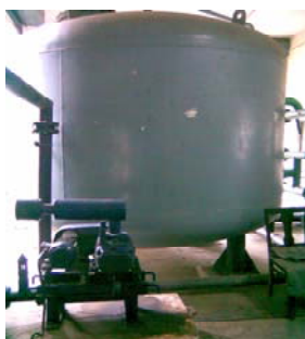
REMOVAL OF FILTER MEDIA FROM PRESSURE SAND FILTER TANK AND SHIFTING TO DRYING BED
