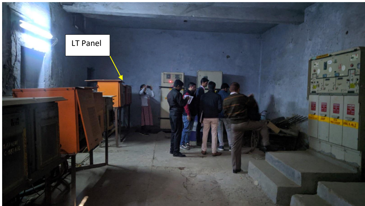
View of complete CR (from entrance)
