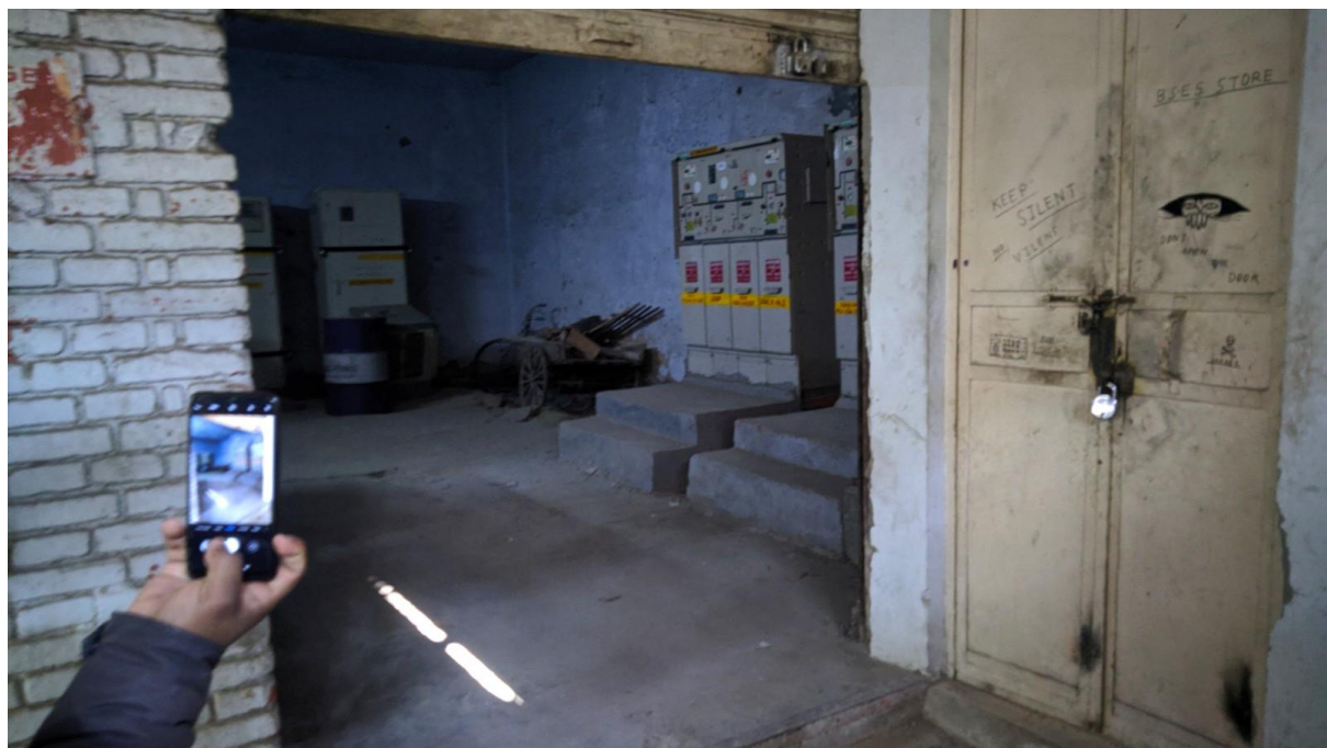
Entry through rolling shutter
