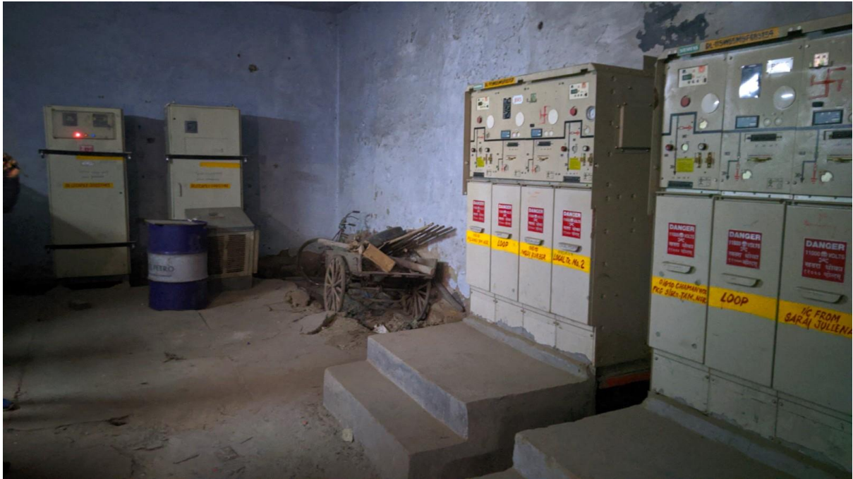
Another view of space for BESS installation
