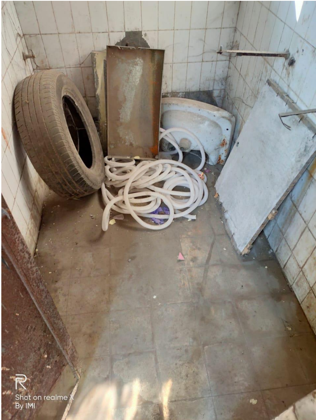
View of space for BESS installation
