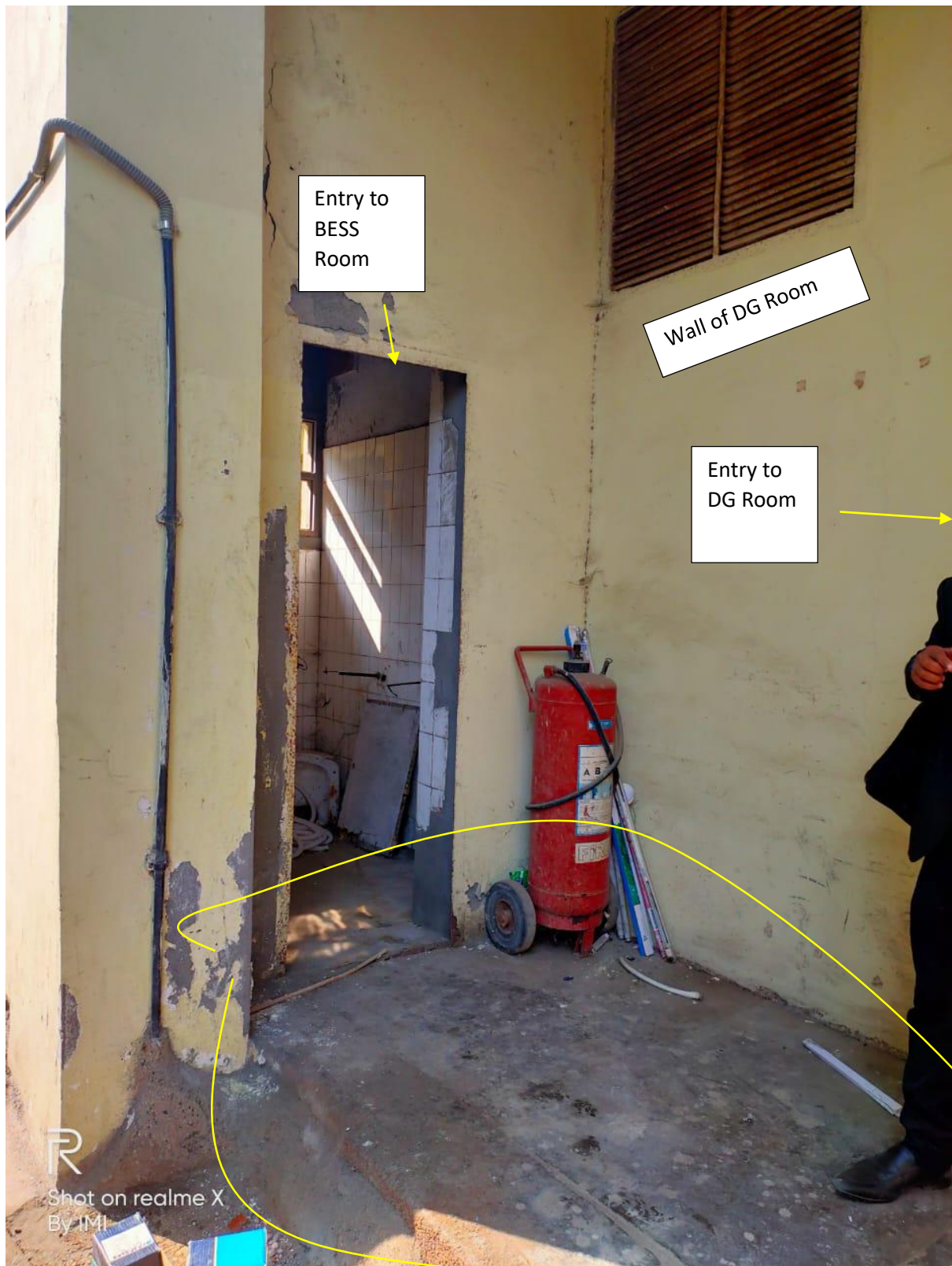
View of space for BESS installation, entry to the BESS room, outside space available for expansion of BESS room
