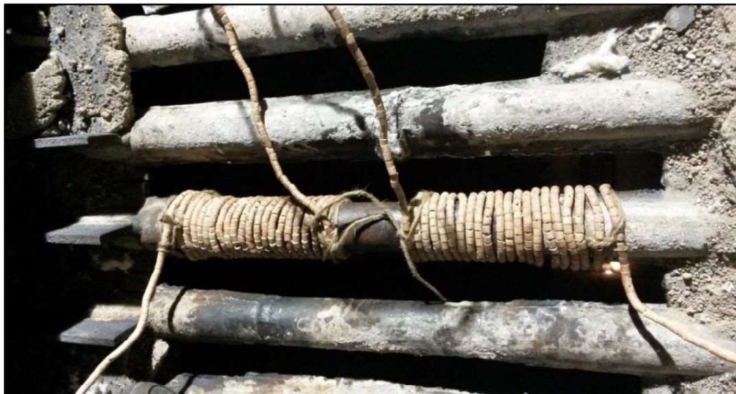
Figure B3.1: Preheating by Resistance coil winding
