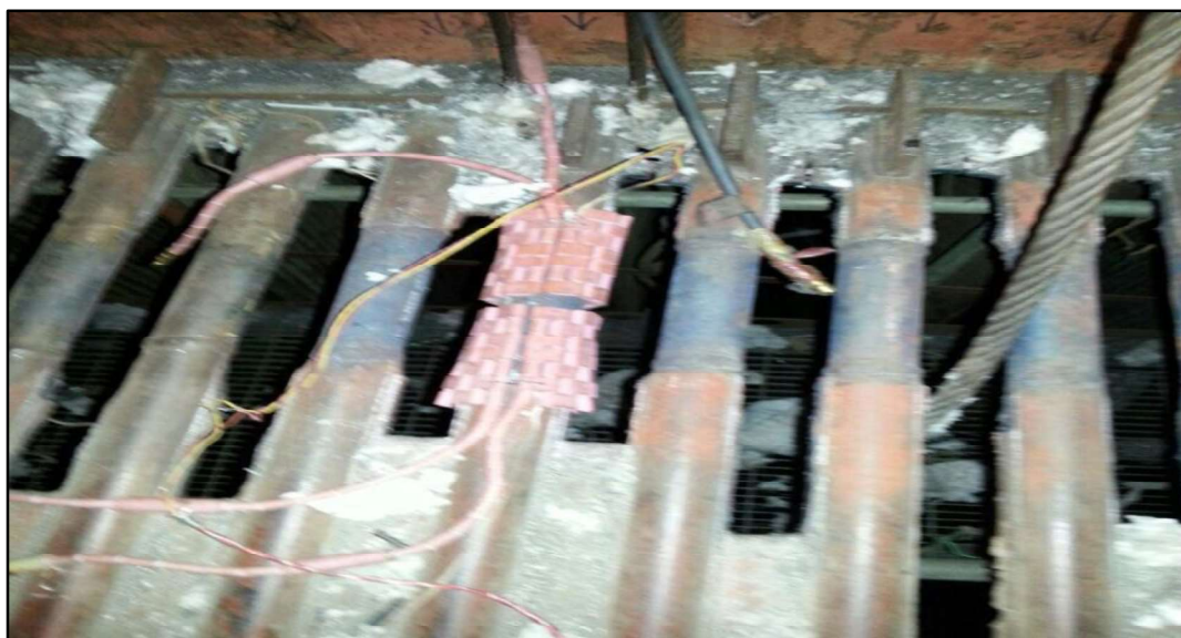
Figure B3.5: Heating pads in place for PWHT
