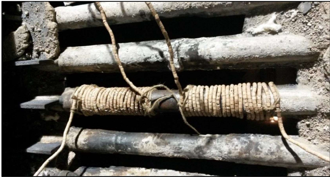
Figure B3.1: Preheating by Resistance coil winding
