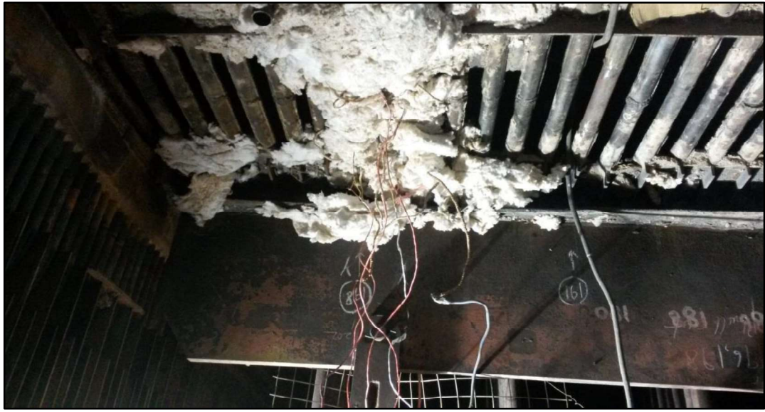
Figure B3.6: PWHT in progress
