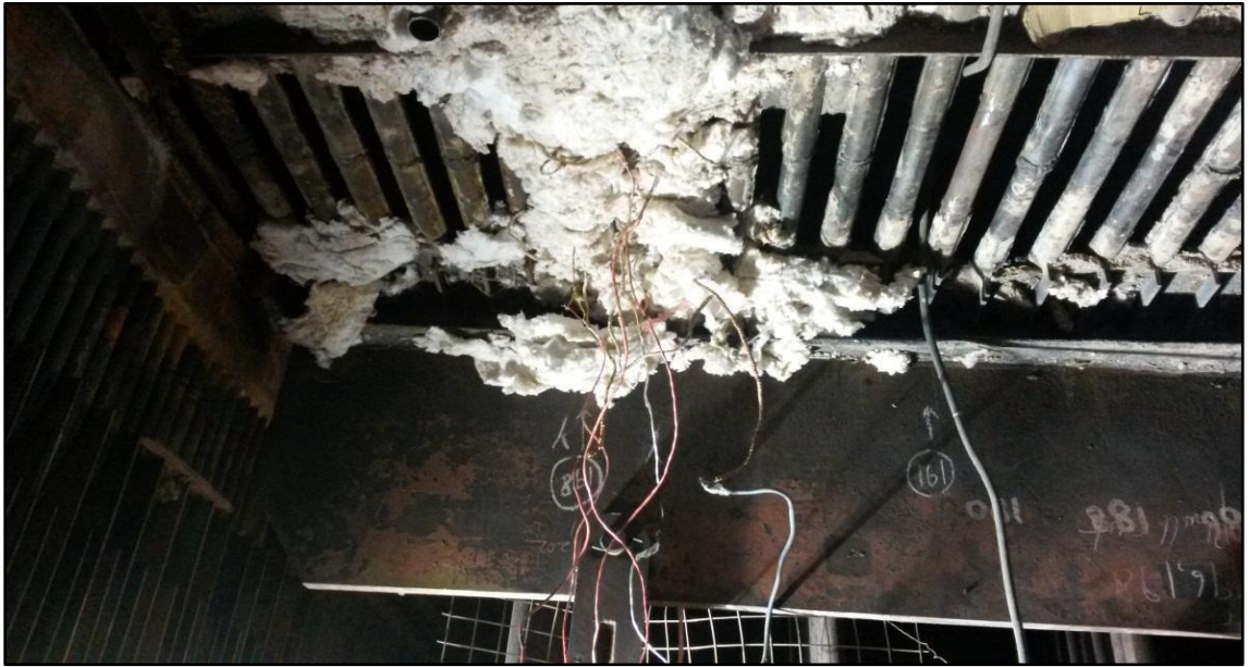
Figure B4.6: PWHT in progress
