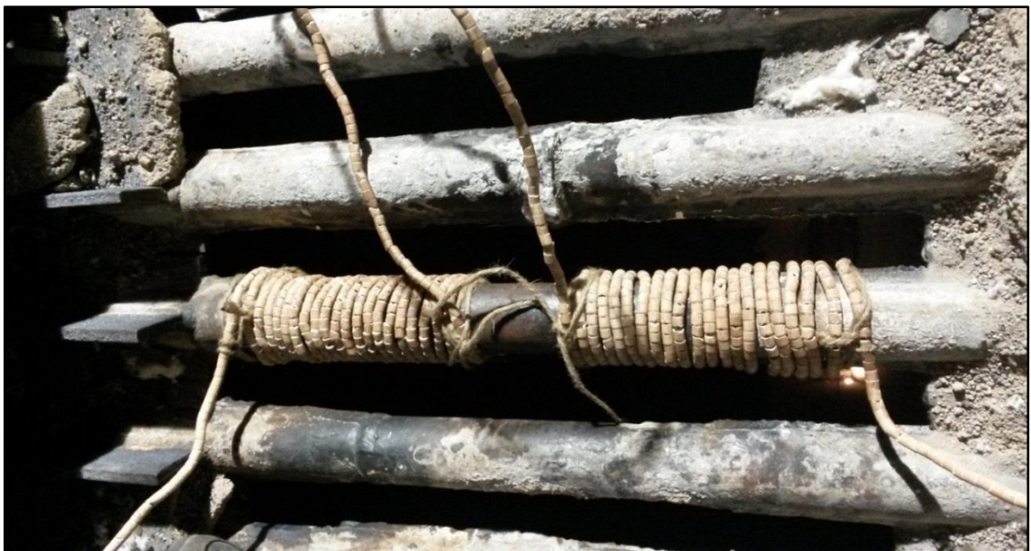
Figure B4.1: Preheating by Resistance coil winding
