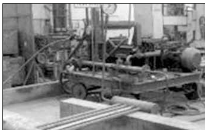
Figure 19 -Hydro test of header assembly
