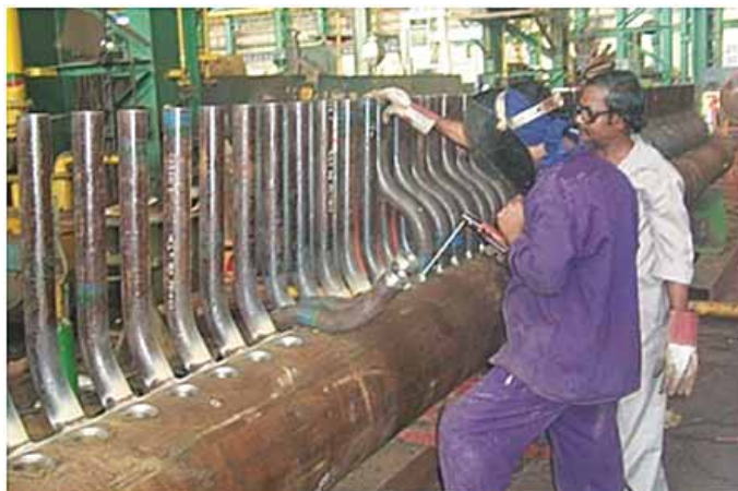
Figure 1 - Manual welding of Header to stub
