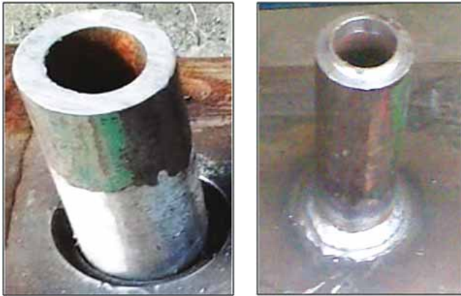
Figure.2 - Edge preparation on header pipe and stub & Stub with complete root pass
