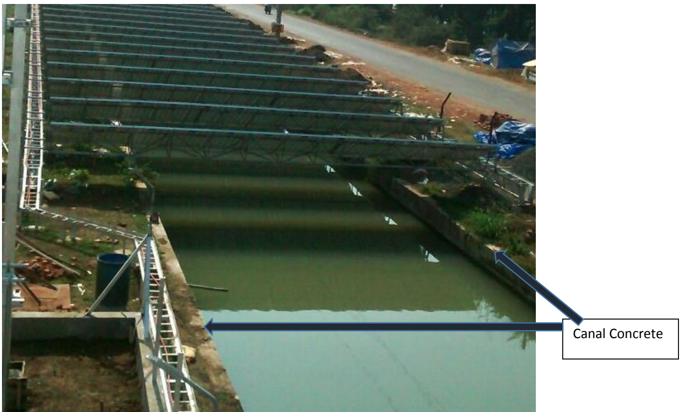
Fig-5: Site during installation stage
