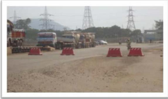
**19.4** When it is not reasonably practical to implement a physical segregation, pedestrians must maintain safety distance of at least 2 meters from moving/operating vehicles at all times.
