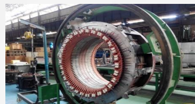
Traction Motor Assembly Facility
