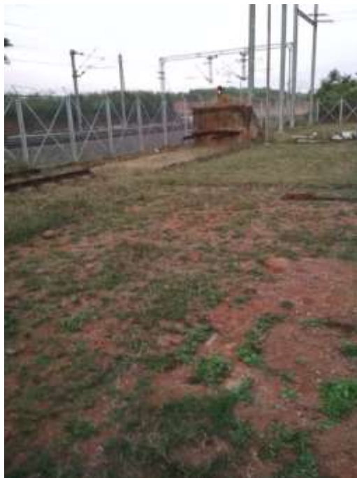
Shimiliguda sub-station photo
