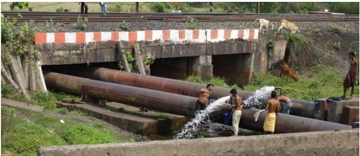
Photo 6.12. Railway culvert over Mundabasti nala. One span carries water supply pipe line
