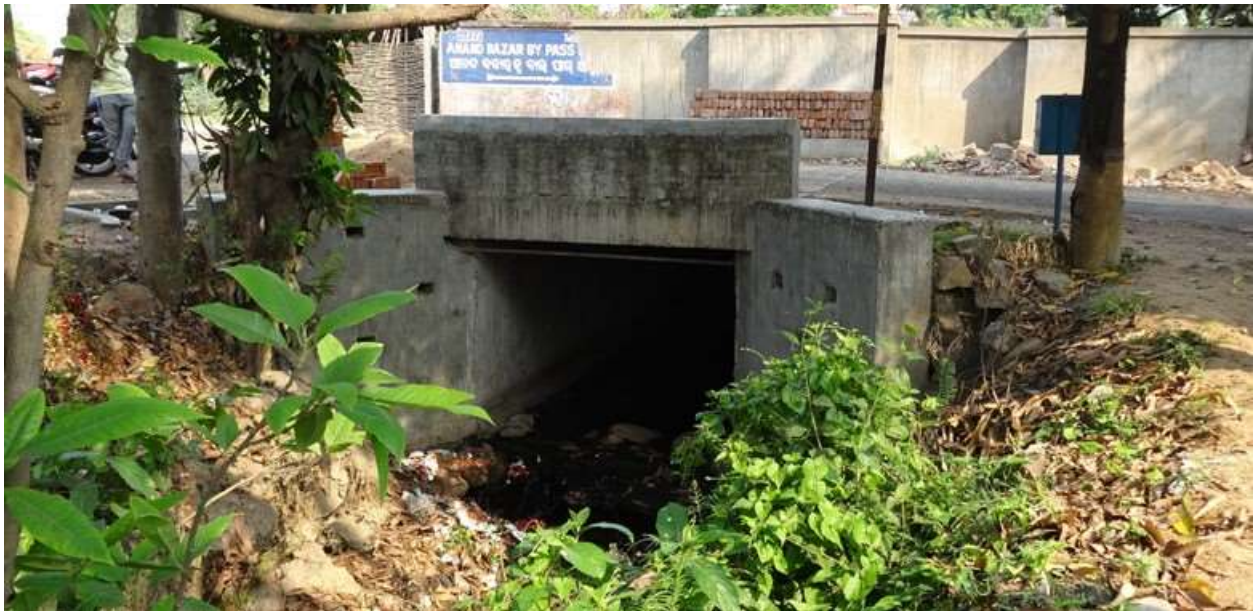
Photo 6.13 Outfall of western trunk drain (OP1) in Nandira nala
