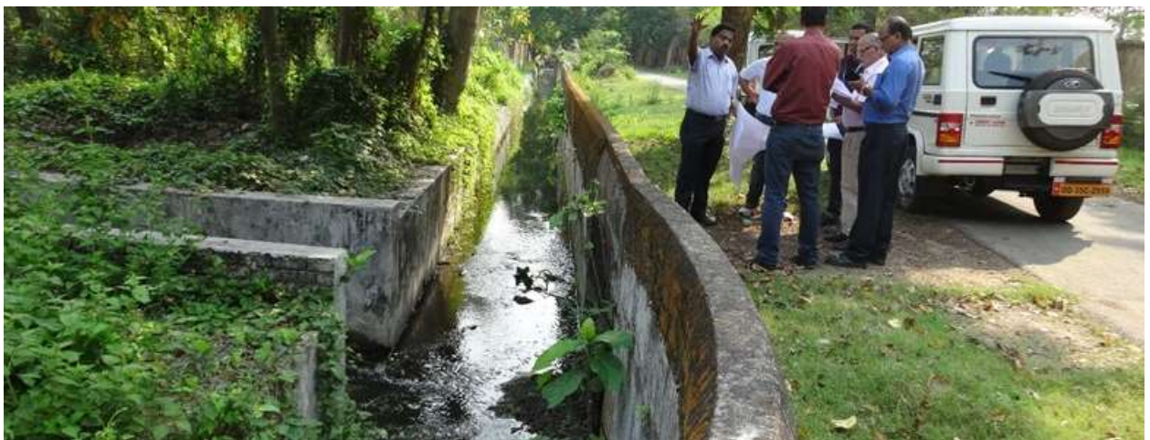
Photo 2.5. Existing drain at OP2
