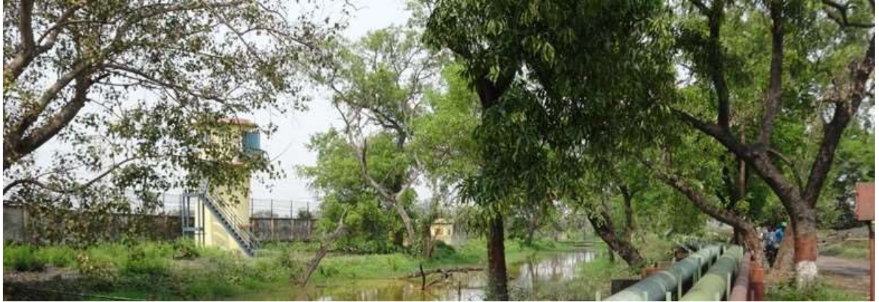
Photo 2.3: Waterlogged area in existing plant area
