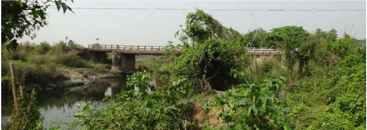
Photo 2.1: Road bridge on Nandiri nala
