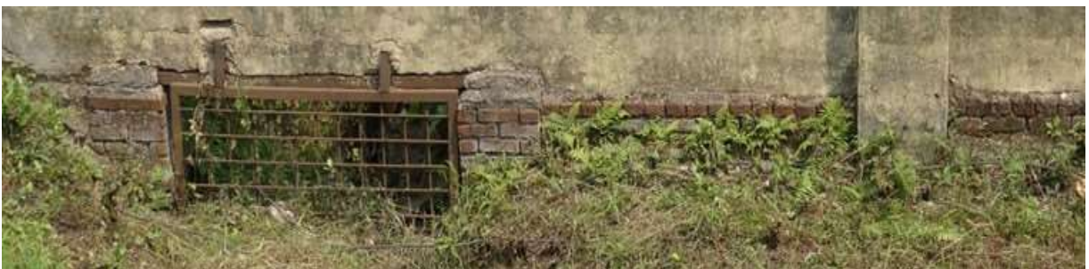
Photo: 6.7 Inlet of Jagannathpur storm water into plant area
