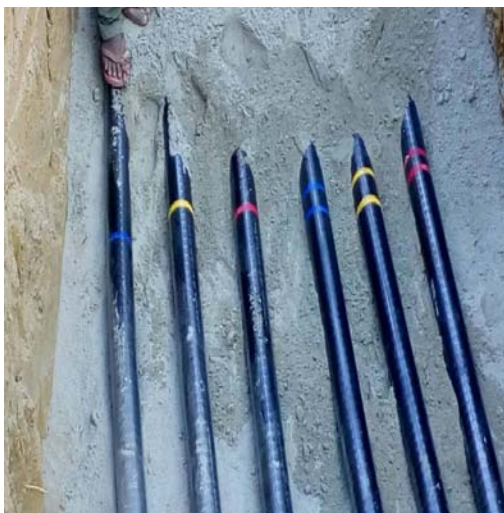
Cable Laying Dressing, Phase Marking, Sand Filling
