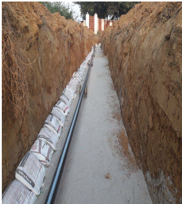
Cable Laying and Protecting with Sand Bags after laying completion, one by one all cables, every time.
