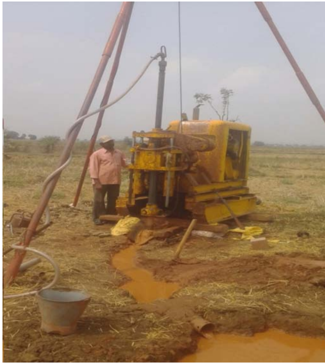
PHOTOGRAPH SHOWING WORK UNDER PROGRESS
