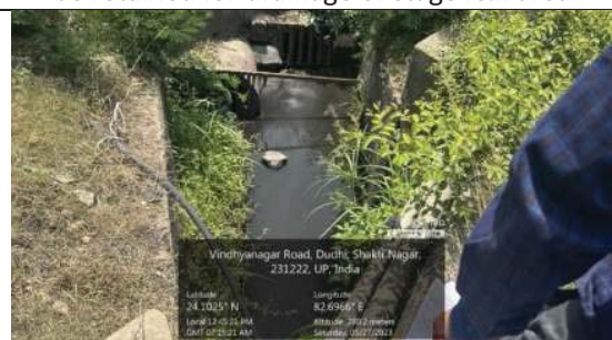
Drain D3- view from outside of boundary wall. This shall be dismantled
