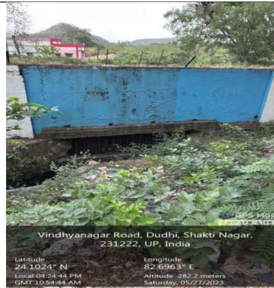
Outfall D3- view from outside of boundary wall
