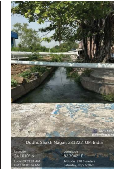
D4 Drain inside plant area. This shall remain for drainage of stagel& II area
