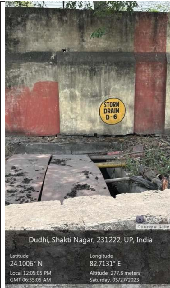
Outfall Drain D6 into Rihand Reservoir-view from inside of boundary wall. This shall be retained for drainage of stage I&II area
