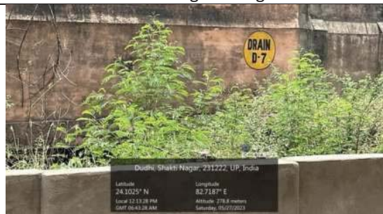
Outfall Drain D7. This shall be retained for drainage of stage I&II area
