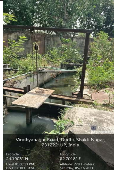
Outfall drain D4- view from outside of boundary wall
