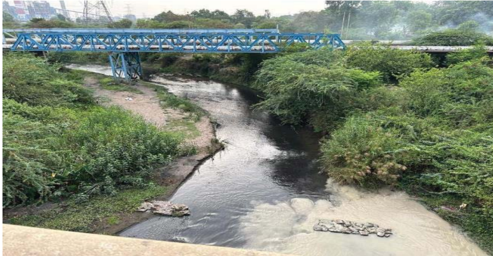
Figure 2.5 Ash slurry flowing into Balina nala due to leakage in the ash slurry pipe –view from road bridge on nala
