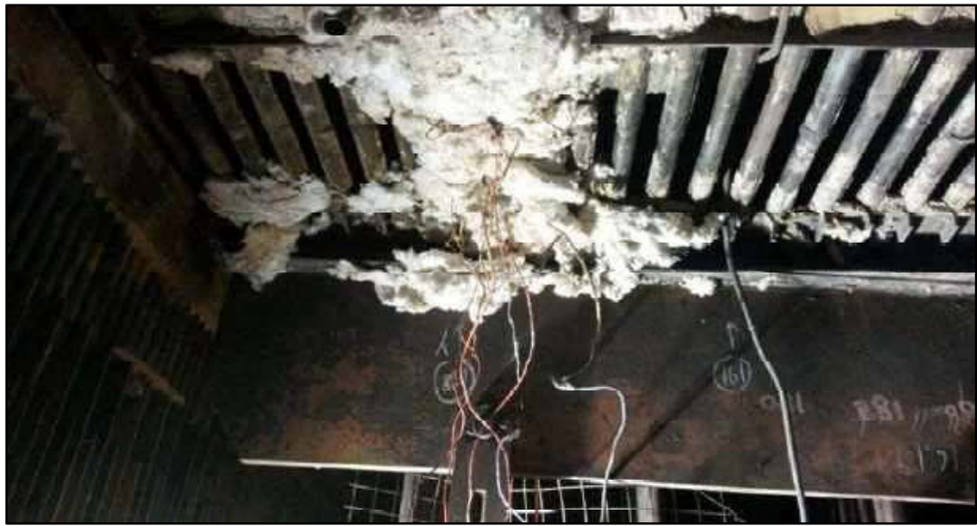
Figure B3.6: PWHT in progress
