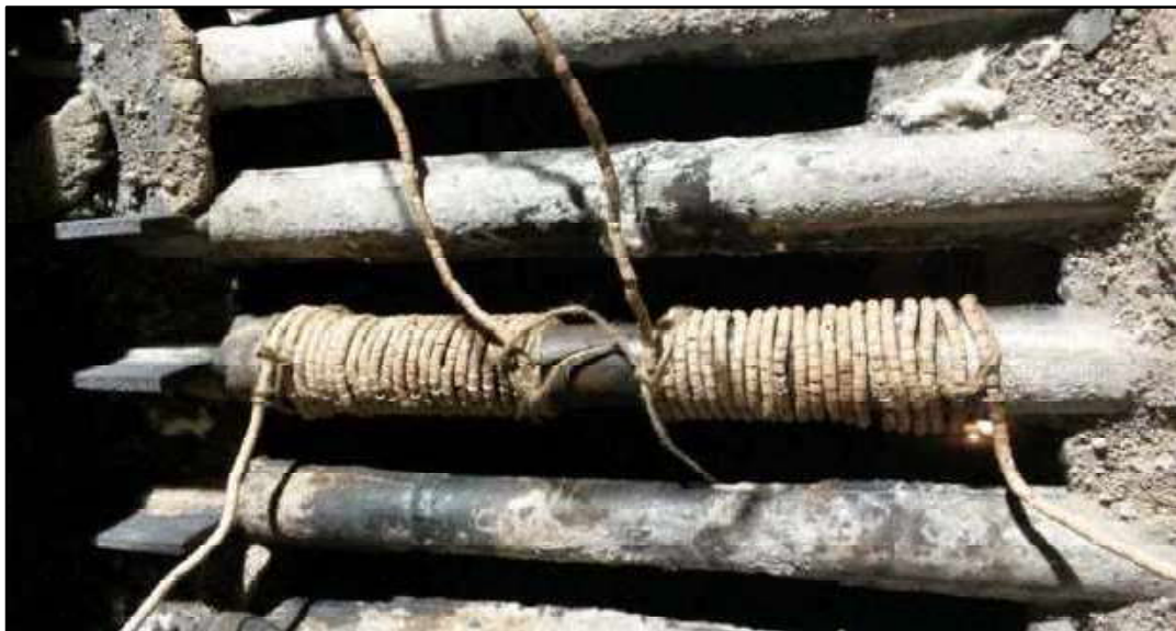
Figure B3.1: Preheating by Resistance coil winding
