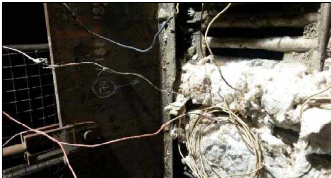
Figure B3.4: Post heating arrangement
