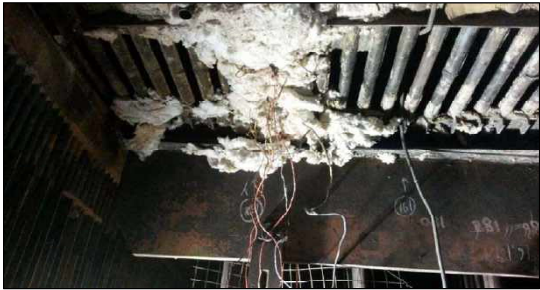
Figure B3.6: PWHT in progress
