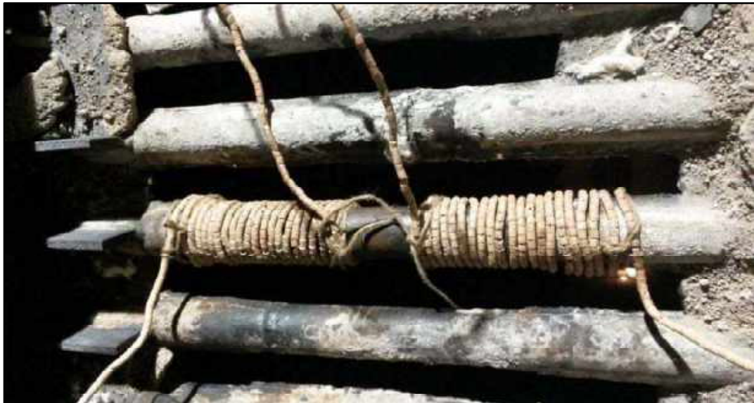
Figure B3.1: Preheating by Resistance coil winding
