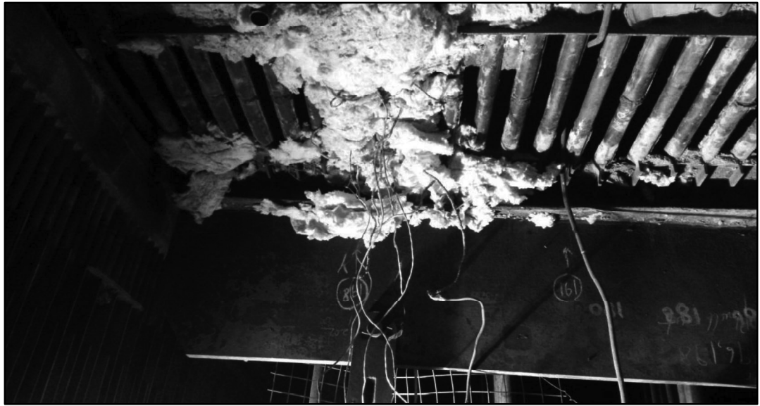
Figure B3.6: PWHT in progress
