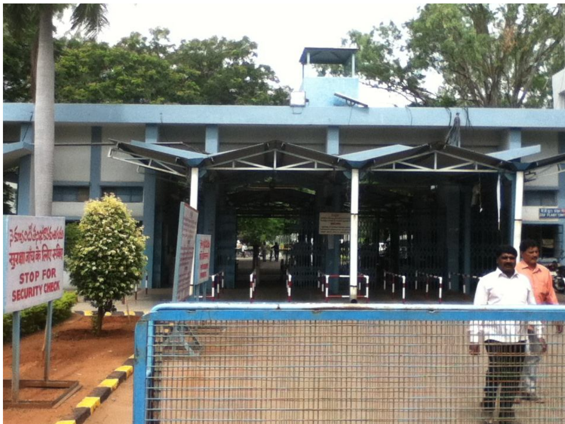
FACTORY MAIN GATE
