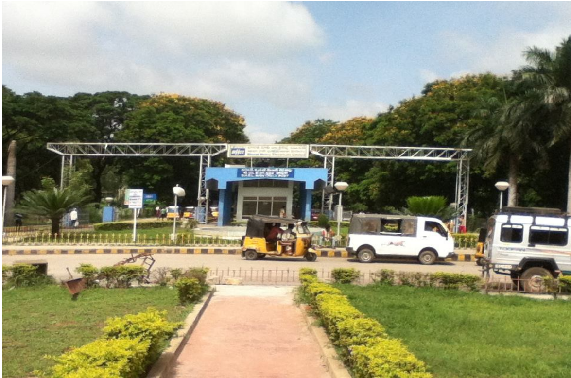
MAIN CHECK POST
