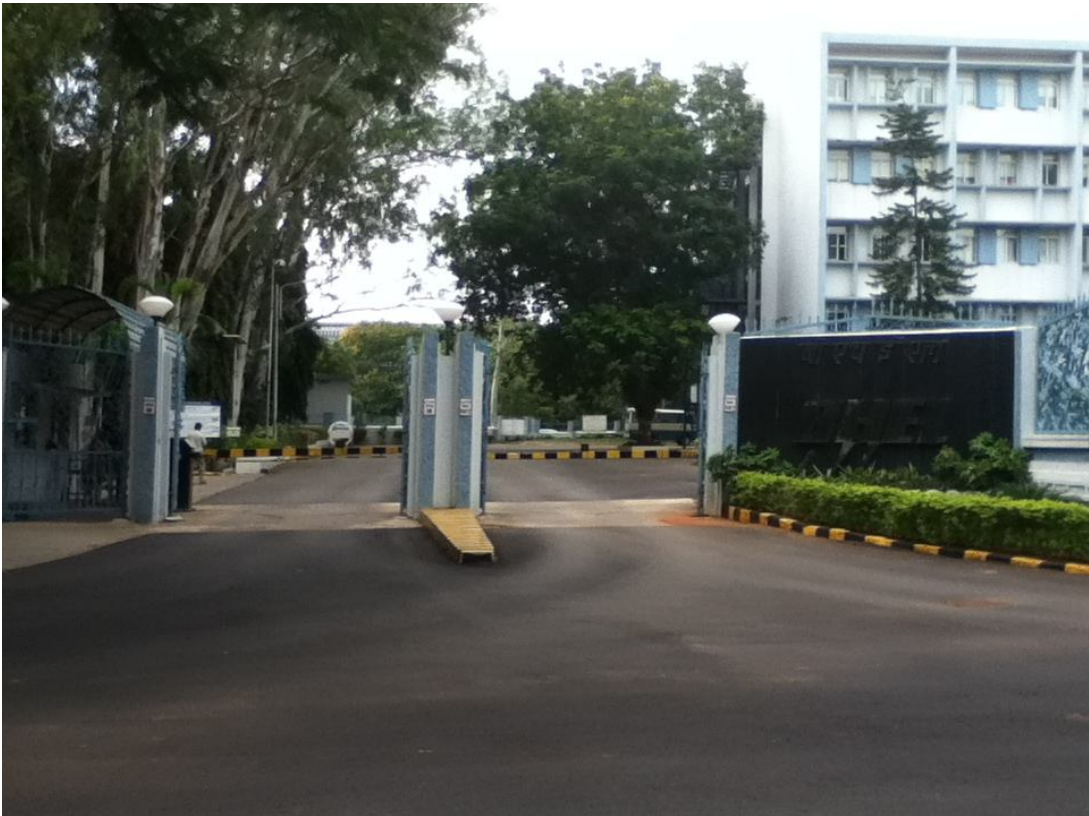
ADMINISTRATIVE BUILDING GATE
