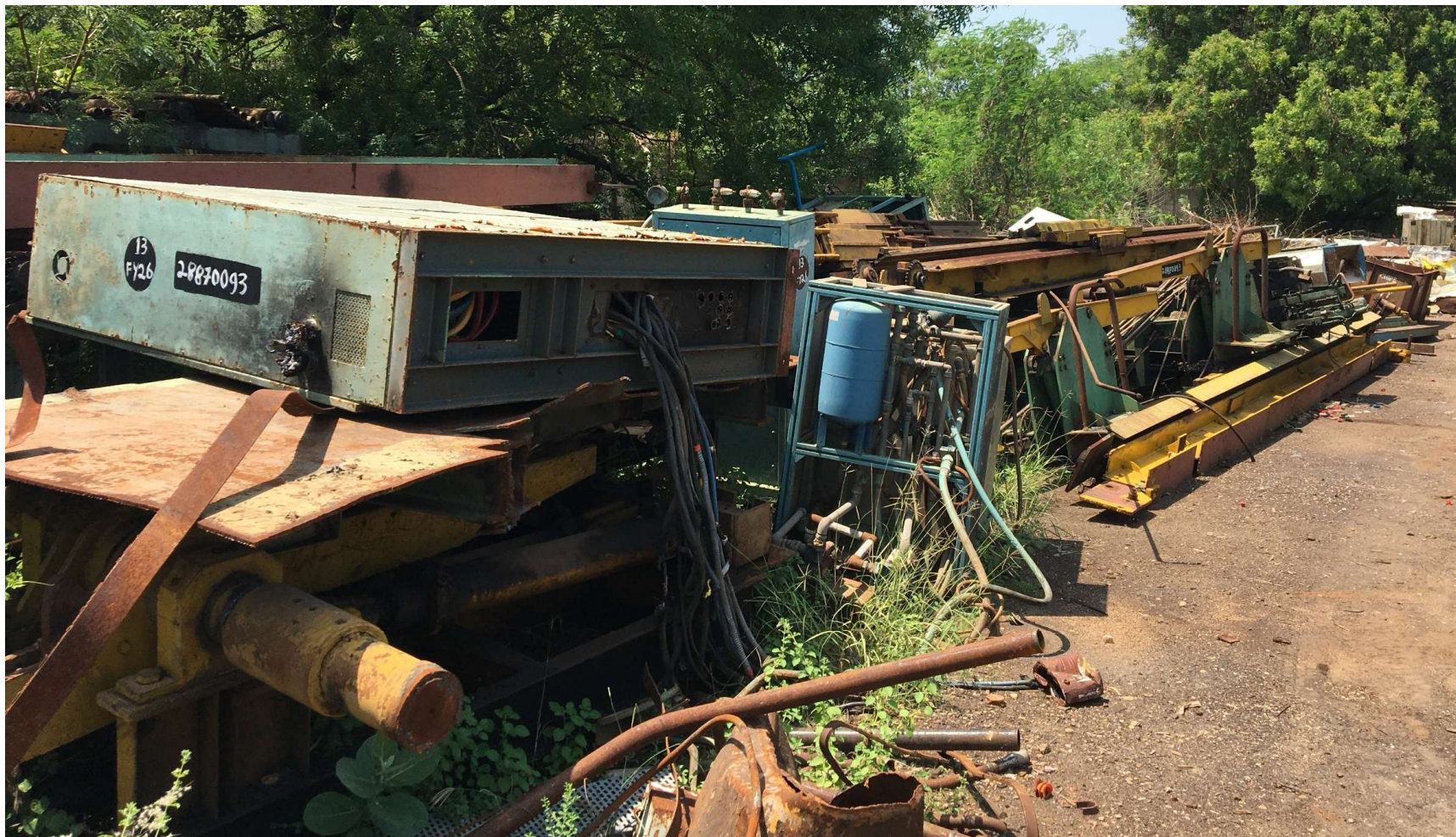
Panel Processing M/C-II (Panle tube to fin welding machine) W.C.NO:2887-0093, YEAR-1975.
