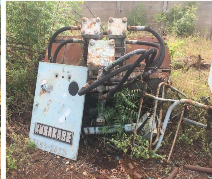
19. SQUEEZING OF SIZING PRESS FURNACE W.C.NO: 3355-2038
