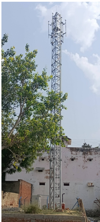
Figure 5: Narrow Based Tower
