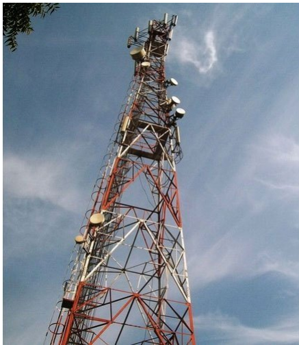
Figure 2: Four Legged Angular Tower
