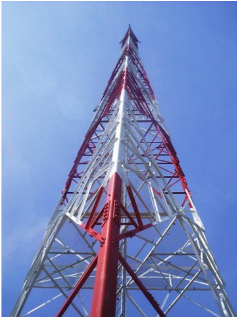
Figure 1: Three Legged Angular Tower
