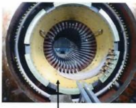
For support and consolidation of the overhang structure of large size TG (above 500 MW ratings).
