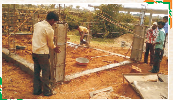
Cremation Ground under construction
