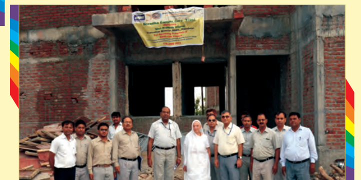
In progress construction of Ganga Prem Hospice
