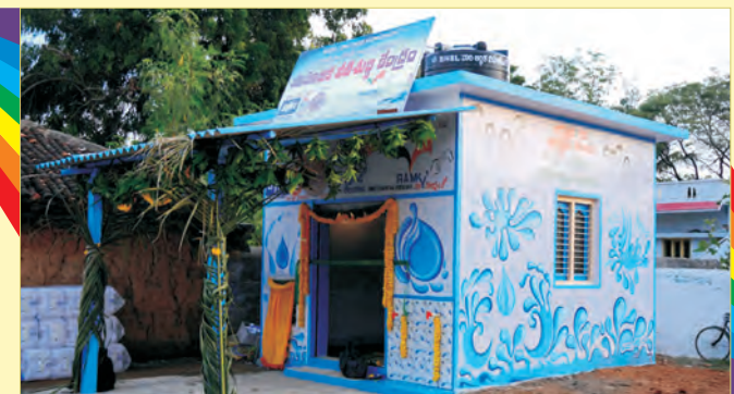
RO Plant at Nalgonda District
