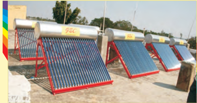
Solar Water Heating System for Telangana state SWRS school/junior college at Hathnoora, Medak district
