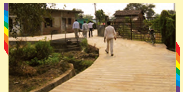
Cement concrete road constructed at a village in Bhandara District, Maharashtra
