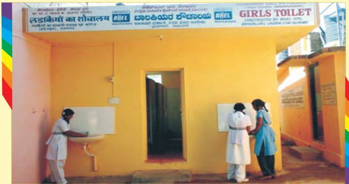
Girls Toilet constructed at Govt. High School, Ramanagar
