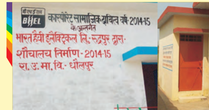
Toilet constructed at Dholpur (Rudrapur)
