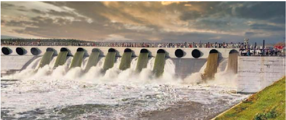
BHEL has commissioned the pumping units of Kaleshwaram Lift Irrigation Scheme (LIS) in Telangana - the world's largest LIS project
