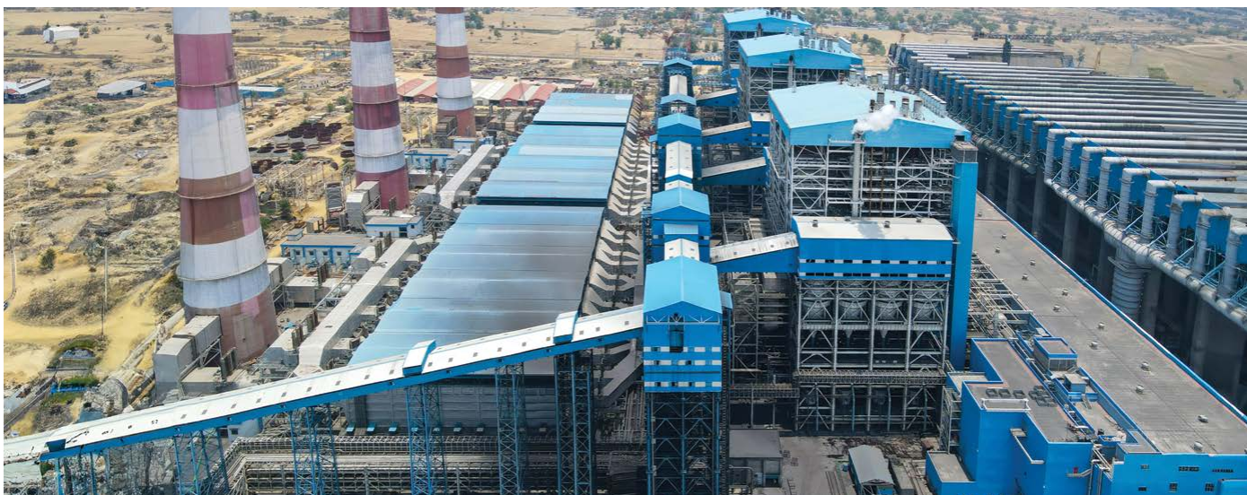
BHEL has commissioned the nation's first utility-scale thermal power plant equipped with Air Cooled Condenser (ACC) at NTPC North Karanpura Super Thermal Power Project Unit-2 (3x660 MW)
