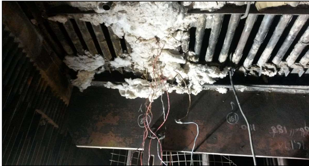
Figure B4.6: PWHT in progress
