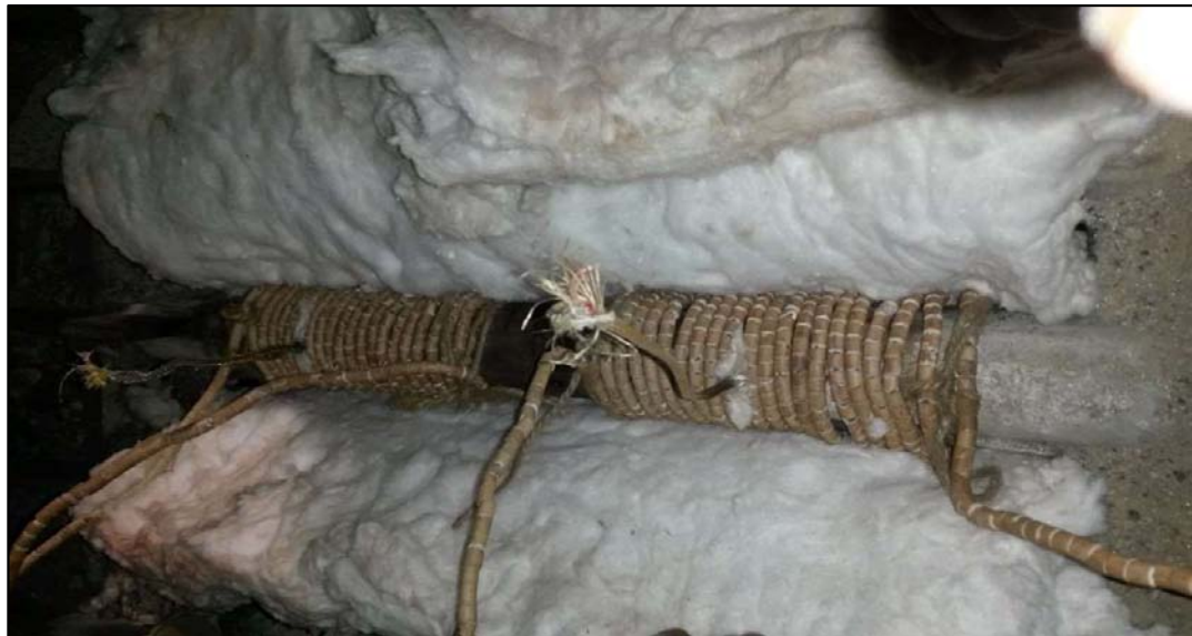
Figure B4.3: Preheating arrangement with thermocouples in place
