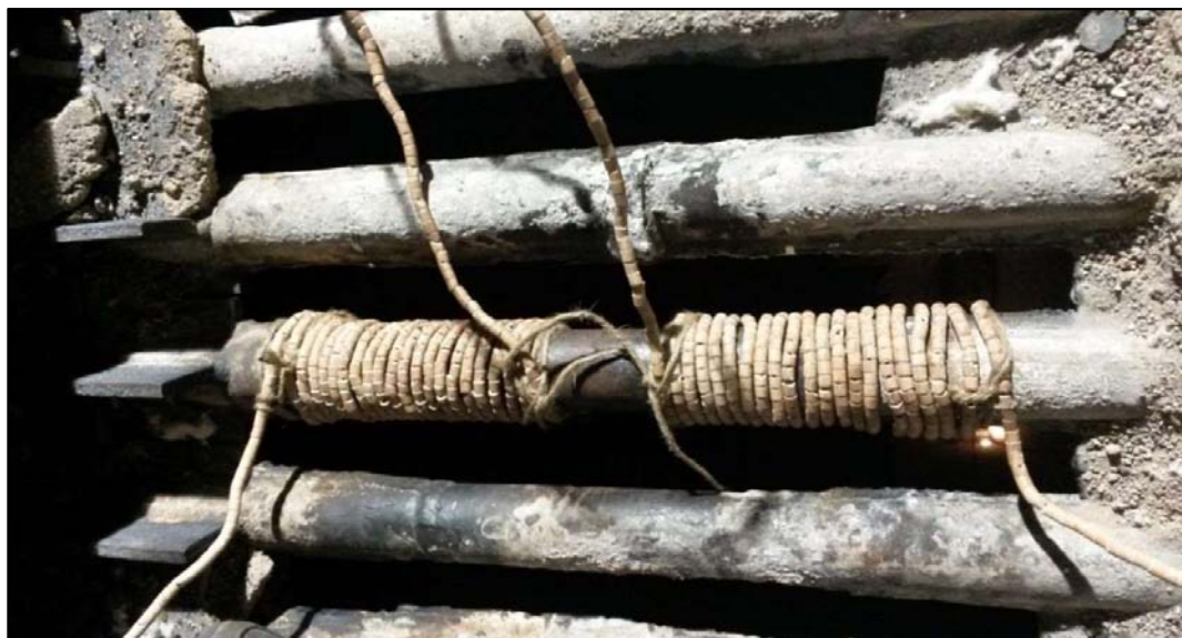
Figure B4.1: Preheating by Resistance coil winding
