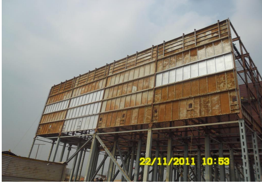
Casing Panel-Being Erected-Unit-2
