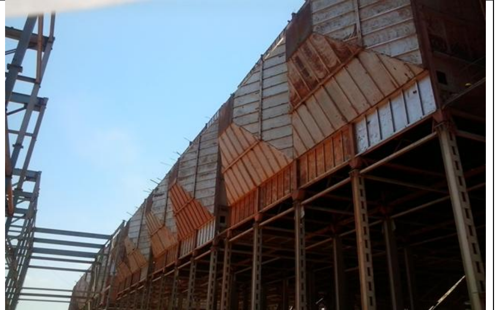
Casing Panel-Subsequently Erected
