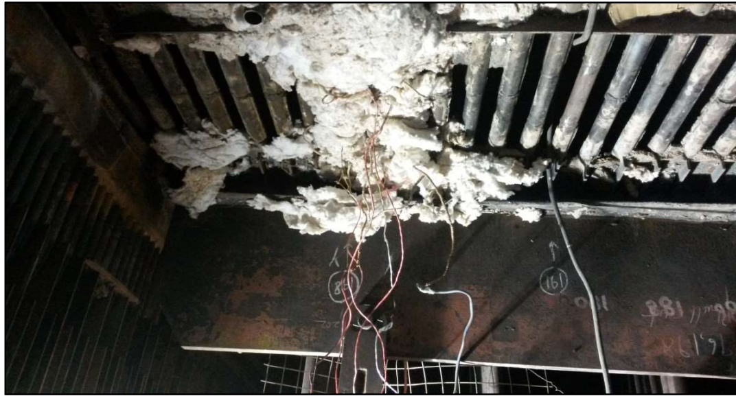
Figure B4.6: PWHT in progress
