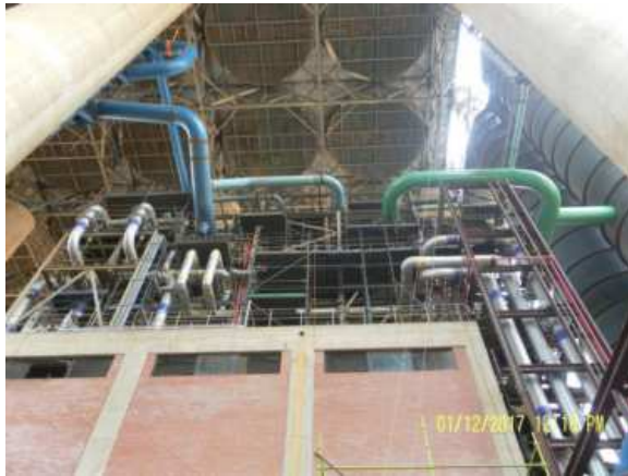
LCM Discharge Line Hotwell – ACC CT
