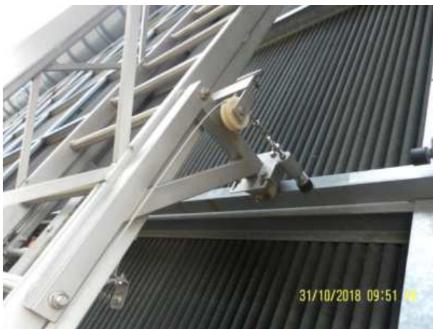
Cleaning ladder brakes
