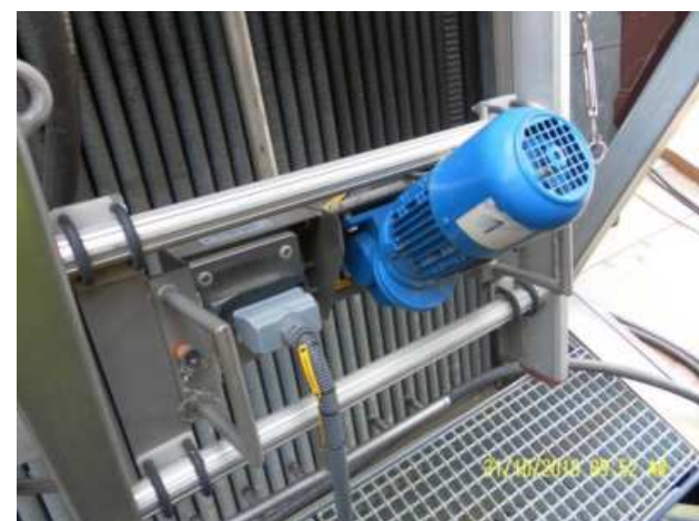
Nozzle beam drive
