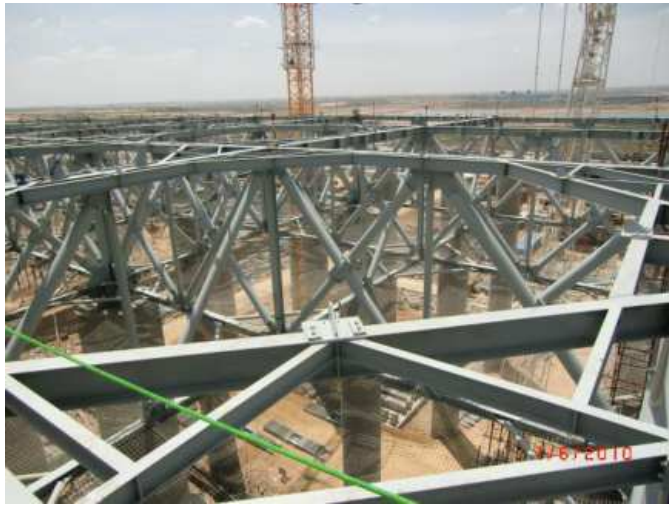
Fan deck Octagonal Beams & Fan Deck Plates Installation
