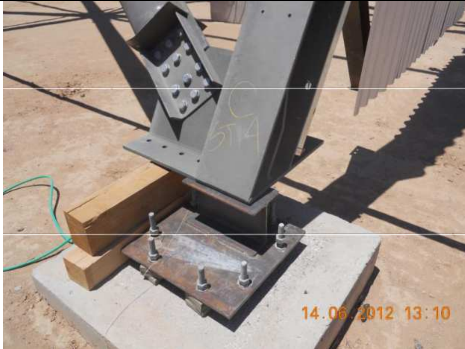
Fabricated Support sitting on the foundation of adjacent street to ensure stable building. Will require additional supporting under the middle cell A-frame
