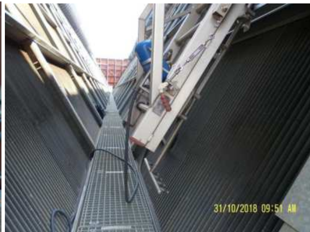
Nozzle beam drive
