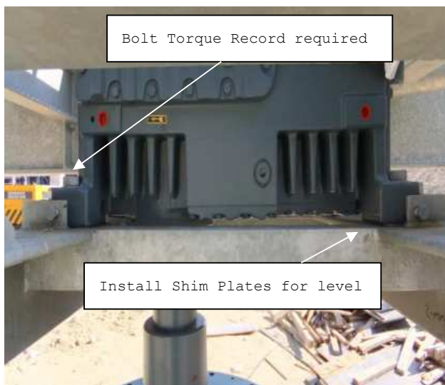
Section 7. Gearbox secured to support frame. Section 7. Fan Hub Plate with blade mounting blocks.
