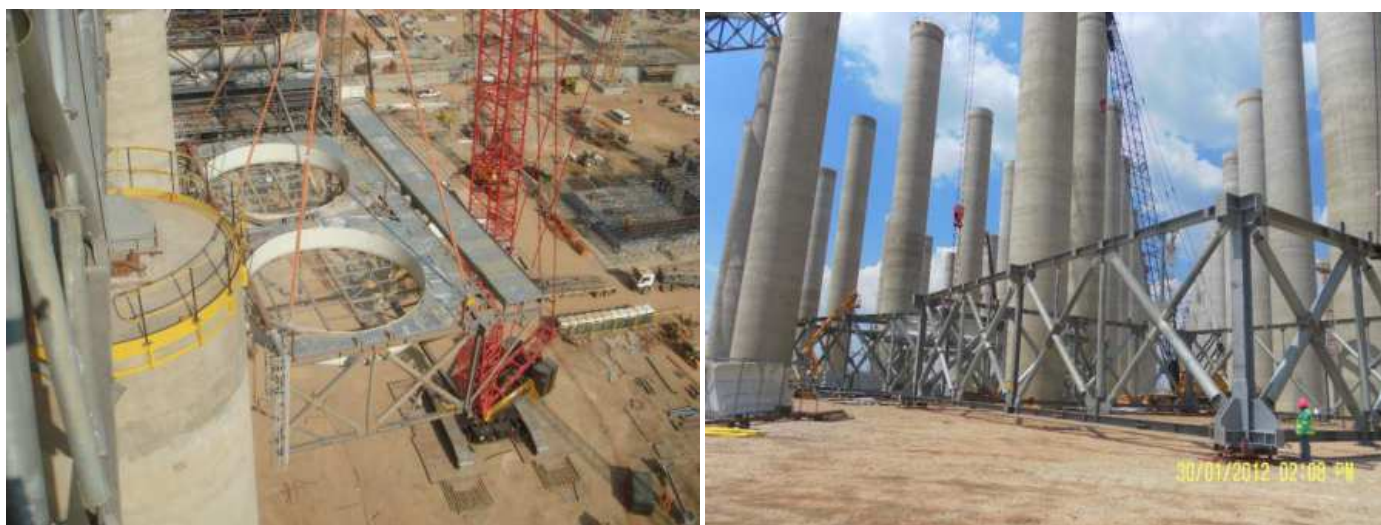
Condensate drain piping LCA-Fan Stack- Fan Deck Beams-Fan Deck Plates Installed onto modules
