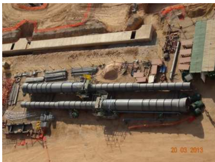
SDM Site assembly to large spools & Installation
