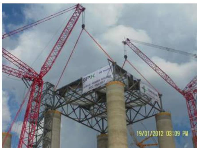
Cantilever module W=57Ton Single Lift CW 450 Tons
