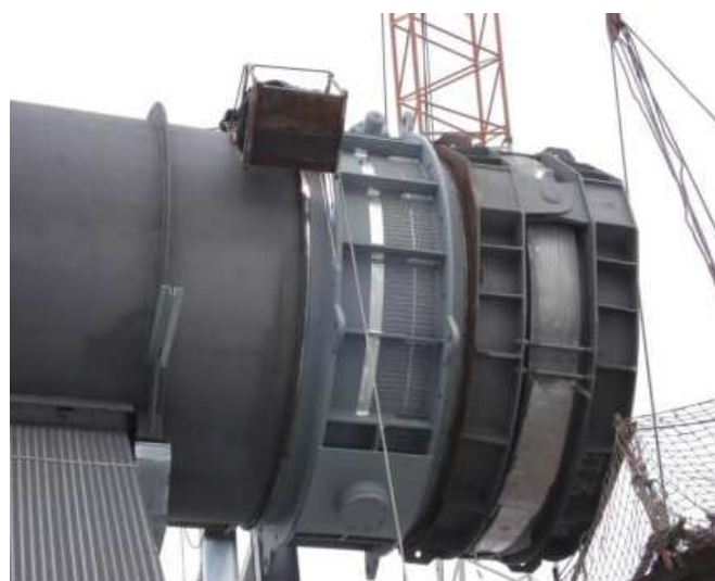
Lifted – Installed Bellow and Valve as one Spool
