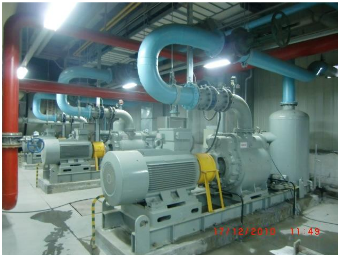
Installed similar Vacuum skid for reference
