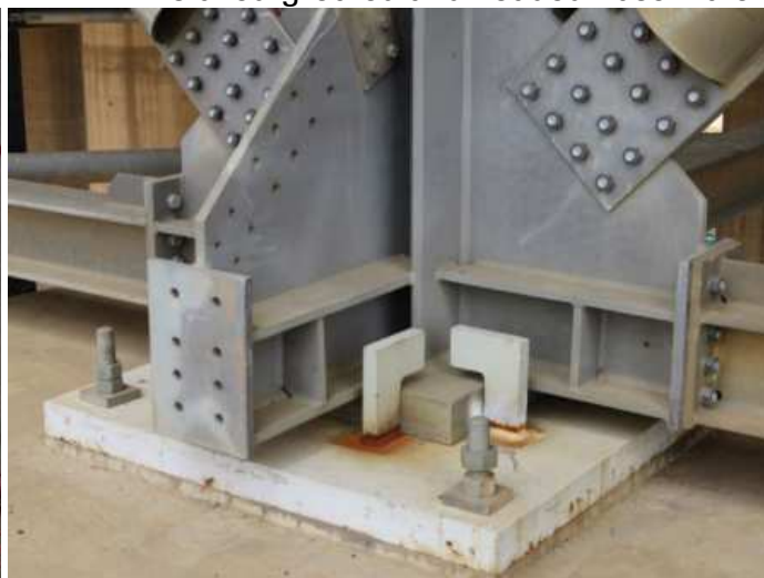
Installed-grouted and Loaded Base Plate
