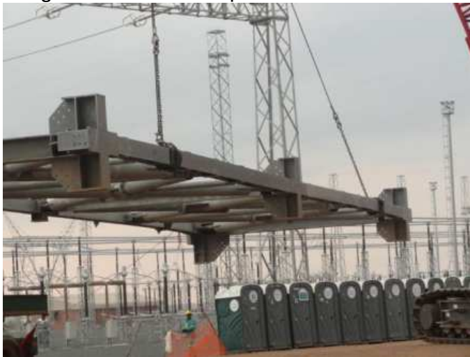
Single Under structure panels installation
