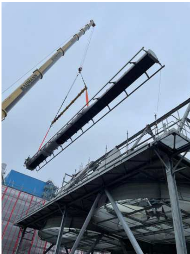
PRE-ASSEMBLED SDM-TSH Covering two Cell with installed BFLY Valve and Cleaning Ladder Top Rails
