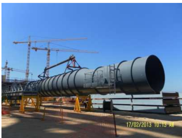
PRE-ASSEMBLED SDM-TSH Covering two Cell with installed BFLY Valve and Cleaning Ladder Top Rails
