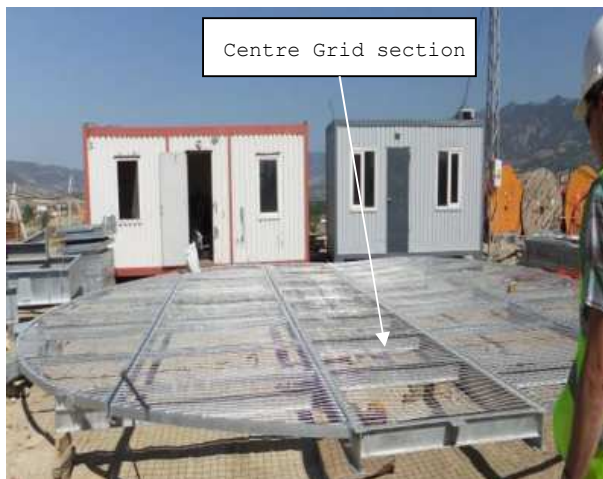
Section 6. Assemble of Fan Screen.
