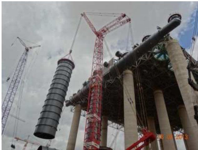
MSED Main Riser Installation W=82 Tons
