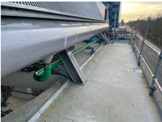
Installed CCM with LCA Drain pipe
