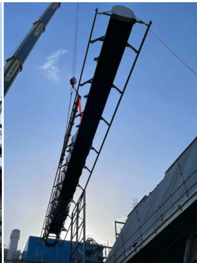
PRE-ASSEMBLED SDM-TSH Covering two Cell with installed BFLY Valve and Cleaning Ladder Top Rails
