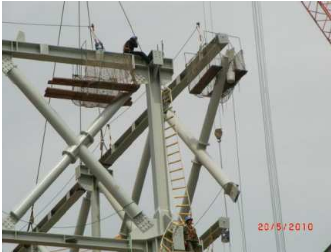
Fan deck Octagonal Beams & Fan Deck Plates Installation
