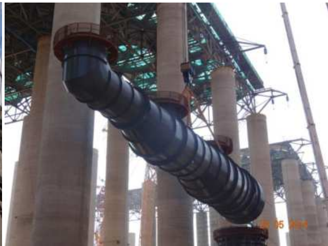
Steam Distribution Manifold Installation W=79 Tons
