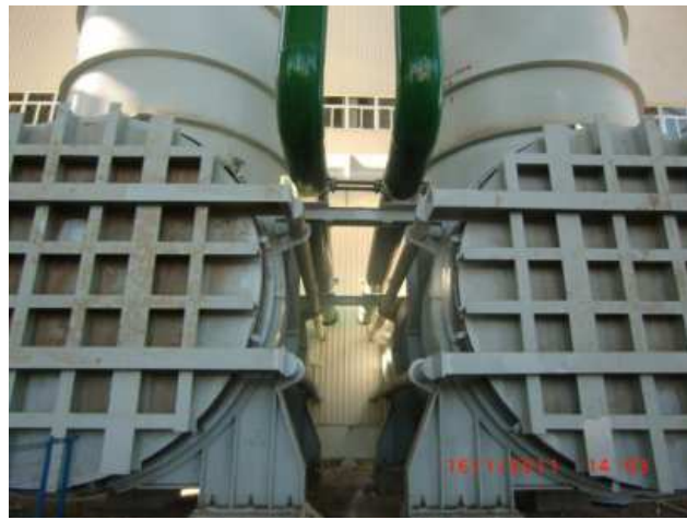
MSED Bottom Elbows -Tee with permanent Blank Plates and Tie Rods
