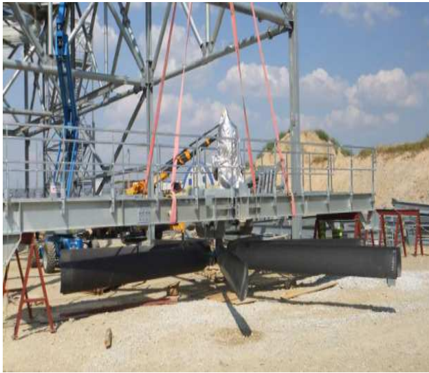
Section 7. Fan Bridge lifting points.
