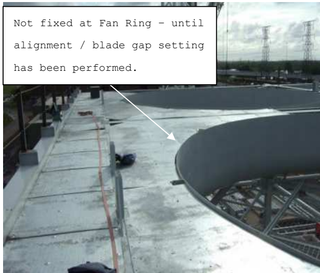
Section 6. Perimeter walk way & Fan Deck Plates. Section 7. Fan Bridge assemble on temporary trestles.
