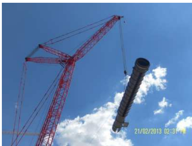
PRE-ASSEMBLED SDM-TSH Covering two Cell with installed BFLY Valve and Cleaning Ladder Top Rails
