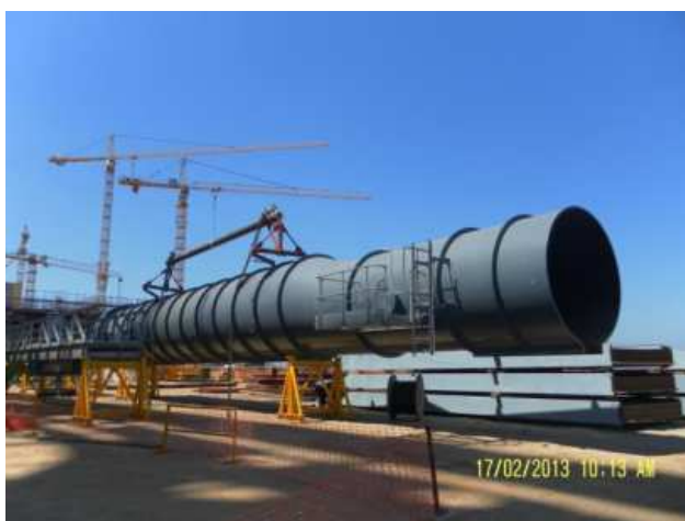
PRE-ASSEMBLED SDM-TSH Covering two Cell with installed BFLY Valve and Cleaning Ladder Top Rails
