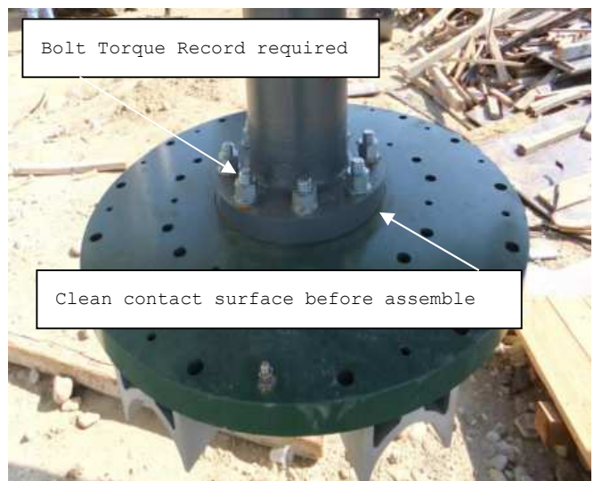
Section 7. Gearbox secured to support frame. Section 7. Fan Hub Plate with blade mounting blocks.
