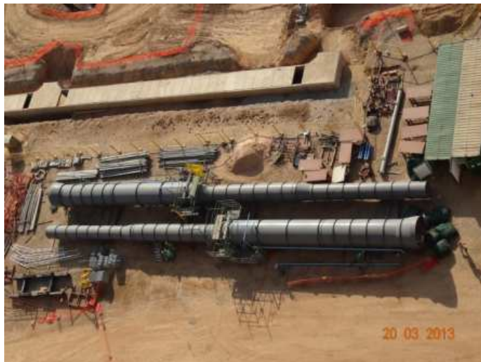
SDM Site assembly to large spools & Installation
