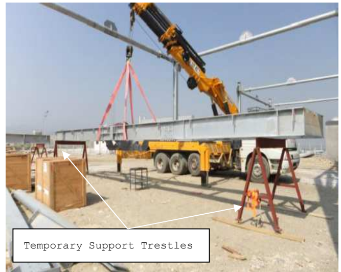
Section 6. Perimeter walk way & Fan Deck Plates. Section 7. Fan Bridge assemble on temporary trestles.
