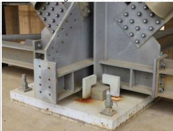
Installed-grouted and Loaded Base Plate
