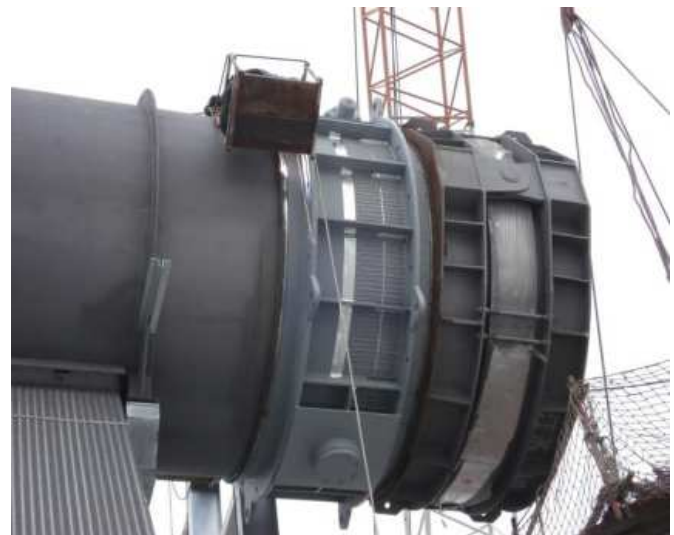
Lifted – Installed Bellow and Valve as one Spool
