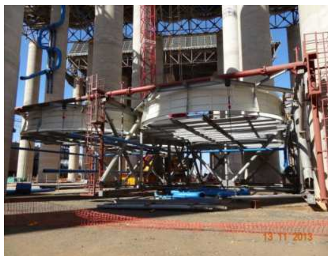
Condensate drain piping LCA-Fan Stack- Fan Deck Beams-Fan Deck Plates Installed onto modules
