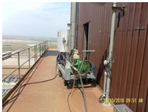
HPP on Transversal walk way
