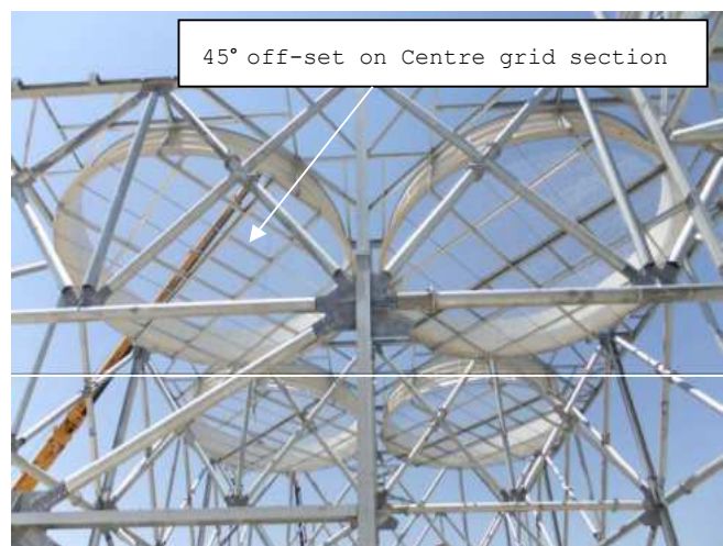
Section 6. Fan Bell's secured onto Fan deck
