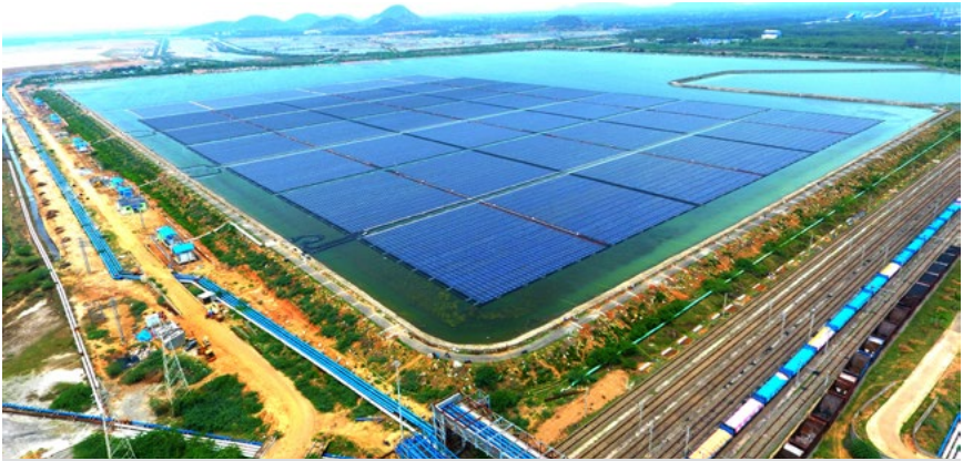
India's largest Floating solar PV Plant (25 MW) commissioned by BHEL at NTPC, Simhadri, Andhra Pradesh
