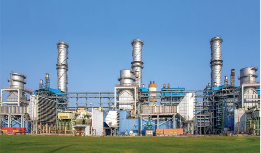
BHEL has made an entry into the downstream oil & gas process package business by securing an order for setting up 525 TPD Sulphur Recovery Unit at IOCL's Paradip Refinery in Odisha
