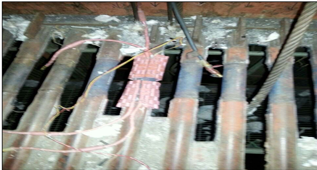
Figure B4.5: Heating pads in place for PWHT
