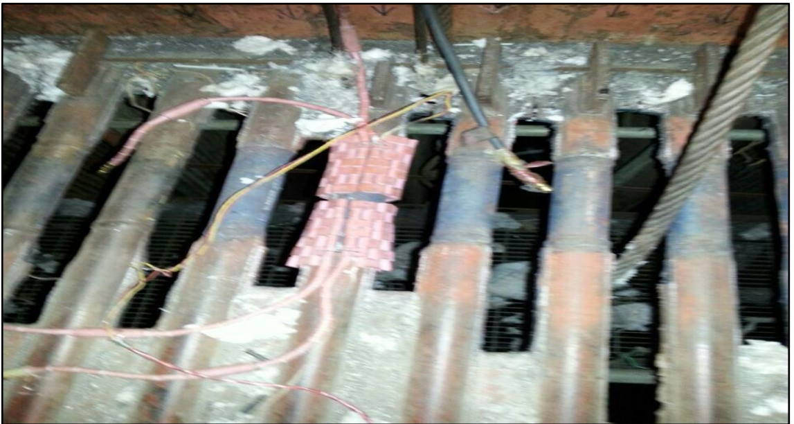
Figure B3.5: Heating pads in place for PWHT
