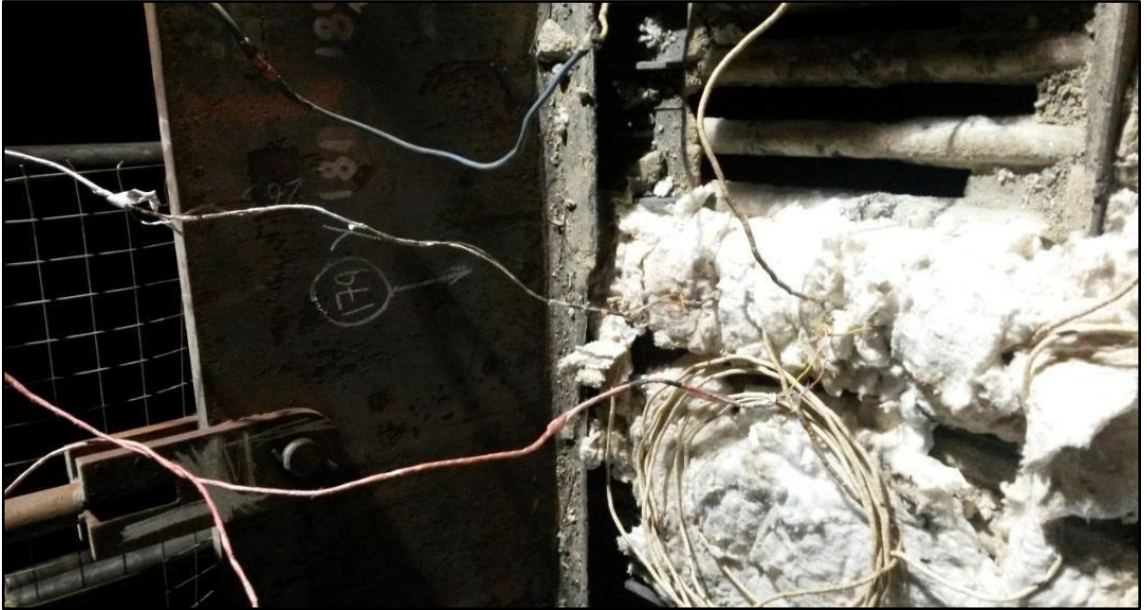
Figure B3.4: Post heating arrangement
